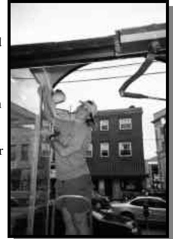
Sara Lowry repairing new display window.
