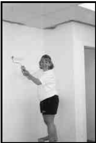
Danielle Carlson sprucing up the new shop.
