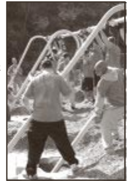
Volunteers complete installation of the swing set.
